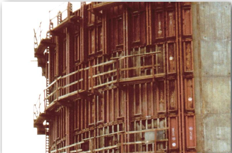
Symons Soldier beams permit bolting on all four flanges in addition to end and web bolt holes. The flange holes are a combination of holes and slots at 3" centers to provide dimensional adjustment and flexibility.
