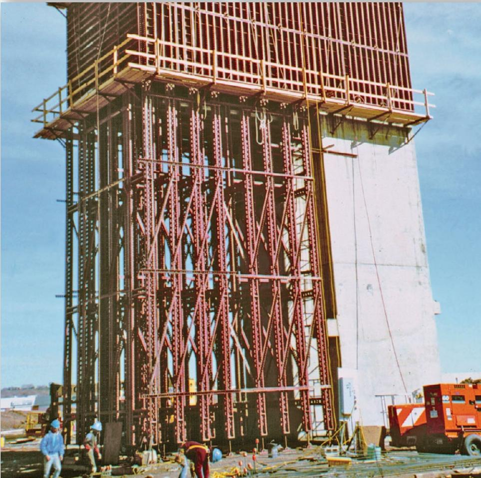
The Symons Soldier system is a lightweight, yet extremely strong, construction beam system that is adaptable to almost any forming or shoring configuration with standard, rentable components and accessories.
